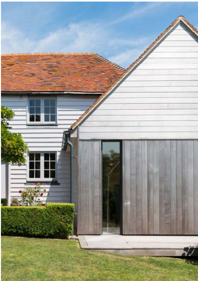
Figure 21: Contemporary example of what could be achieved by referencing clay pantiles and timber materiality of Swarland's local vernacular
