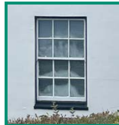
Paned sash windows
