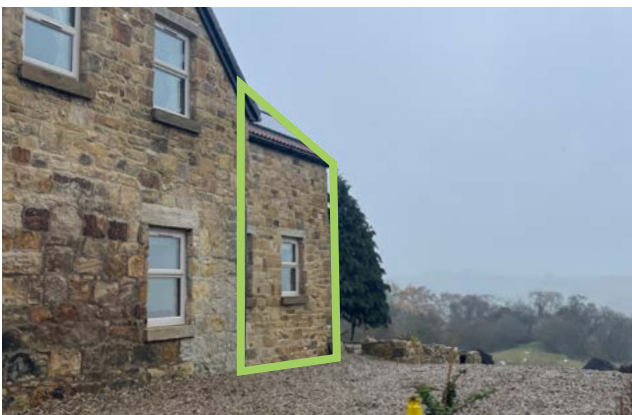
Figure 37: Existing building and new build extension at rear mirroring the gable, materials, and overall design of the original building
