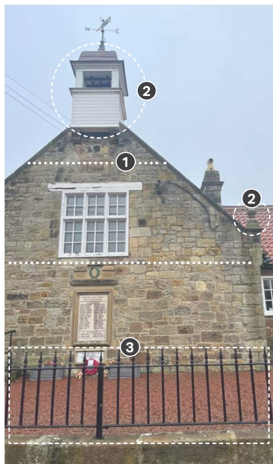
Figure 25: Grade II Listed Jubilee Hall fronting the village's main street
