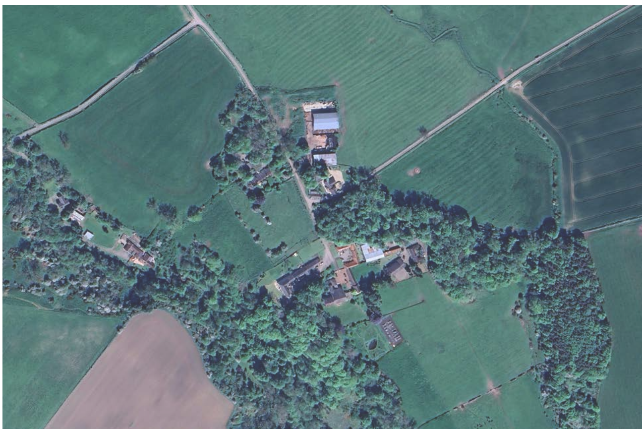
Figure 50: Hazon aerial - cluster of homes and agricultural buildings distributed in an organic layout. Development and planning applications within Hazon will be limited to extensions, conversions and those relating to agricultural use. The hamlets rural character must be preserved by minimising development.
