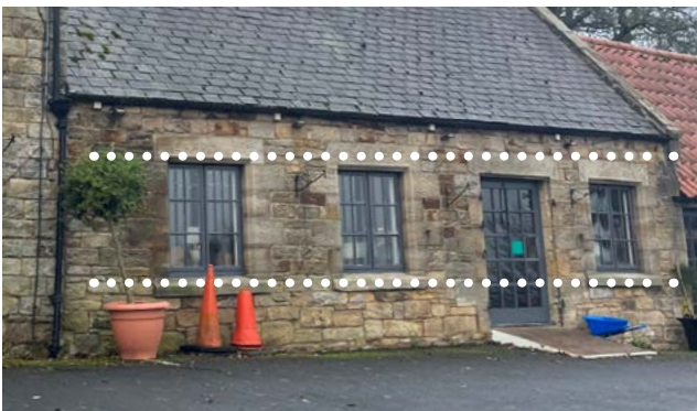
Figure 38: Vertically aligned fenestration and attractive window treatments using panelling and subtle colour
