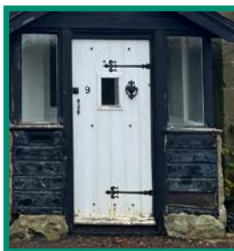
Timber door with wrought iron detail
