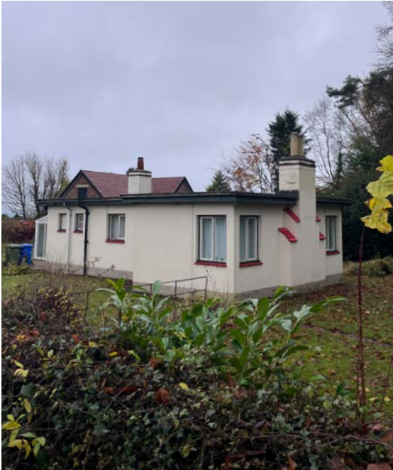
Figure 11: Flat roofed Grade II Listed building fronting Nelson Drive
