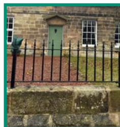
Low limestone wall with wrought iron fence (mostly along the main street and civic buildings)
