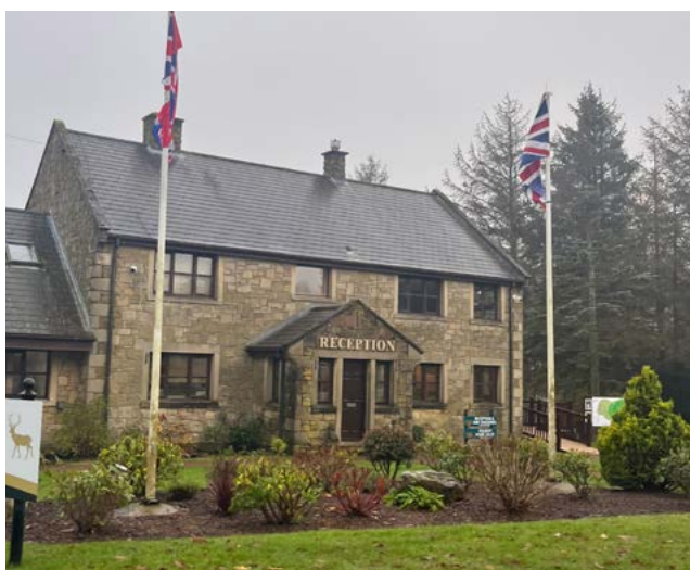
Figure 52: Percy Wood Country Park reception building at its Leamington Lane access
