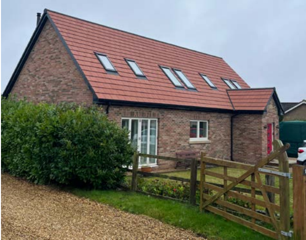
Figure 35: Recent build in Swarland with an attractive frontage (paddock fencing and hedgerow boundary treatment) and use of local materials
