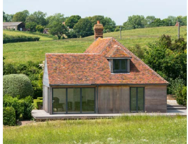
Figure 36: Contemporary example of how new development can reference the build, style and materials of the area's historic buildings
