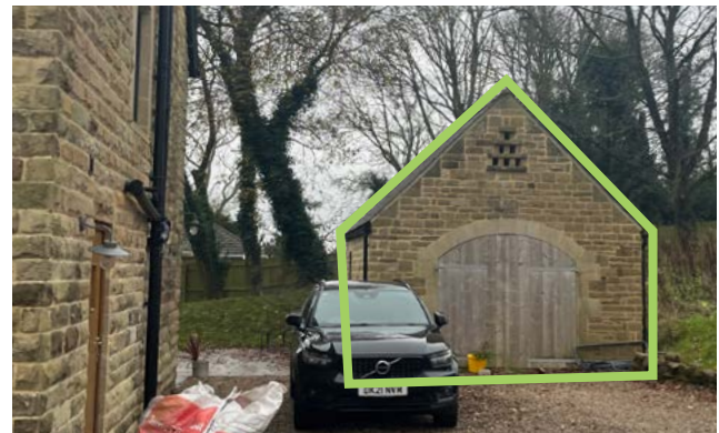
Figure 22: North Lodge garage - new build garage of North Lodge harmonising with the main dwelling by incorporating character detailing from North Lodge
