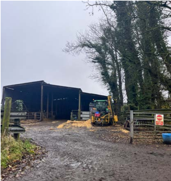
Figure 44: Agriculture infrastructure, Hazon
