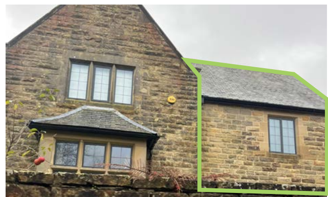
Figure 23: North Lodge extension - new build extension harmonising with the materials and style of the original lodge building
