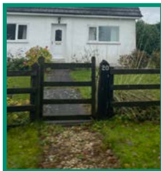
Timber paddock (open board horizontal) fencing and gates
