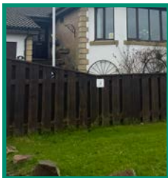
Vertical open board fencing
