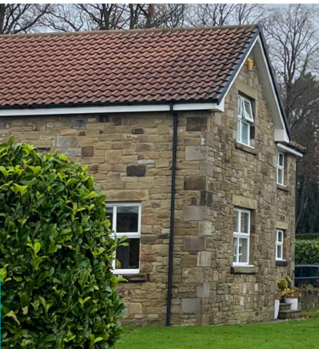
Figure 61: Recent development in Swarland reflecting local heritage and character with its limestone facade, red clay pantile roof and limestone quoins, window headers and cills.
