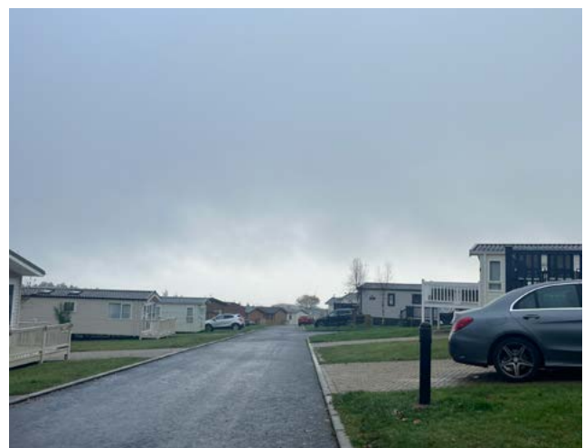
Figure 57: Percy Wood is a large caravan holiday park with connecting roads running throughout it
